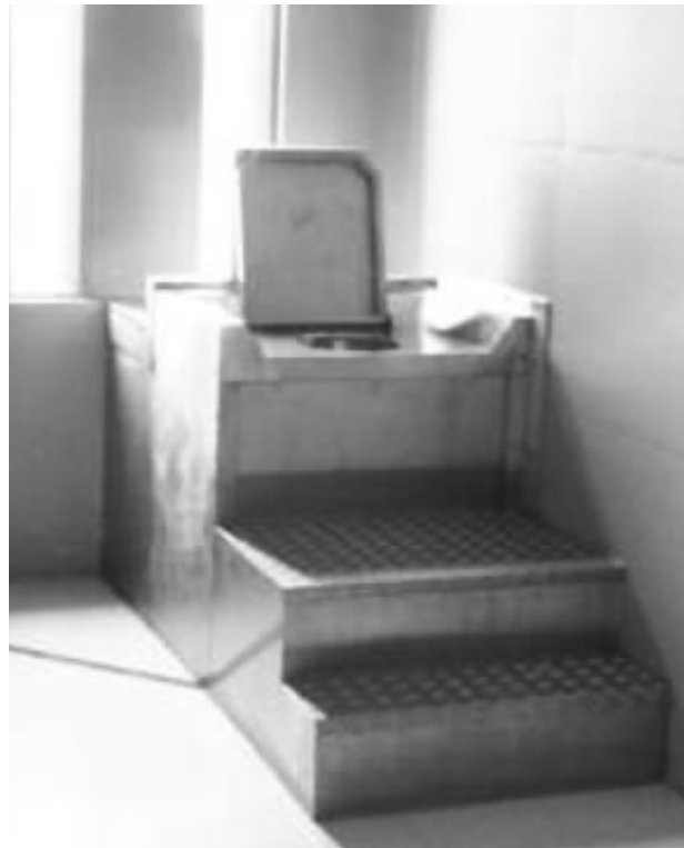
A "dry cell" toilet
