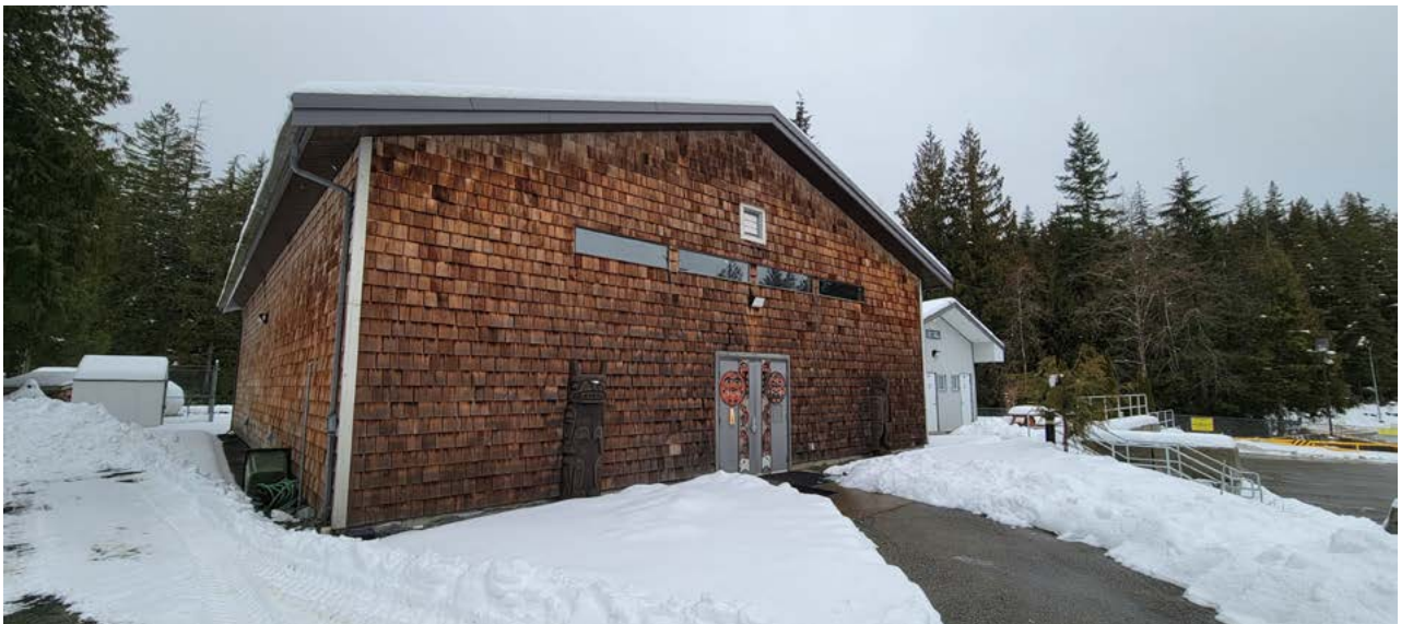
Exterior of the longhouse at Kwikwèxwelhp Healing Village
