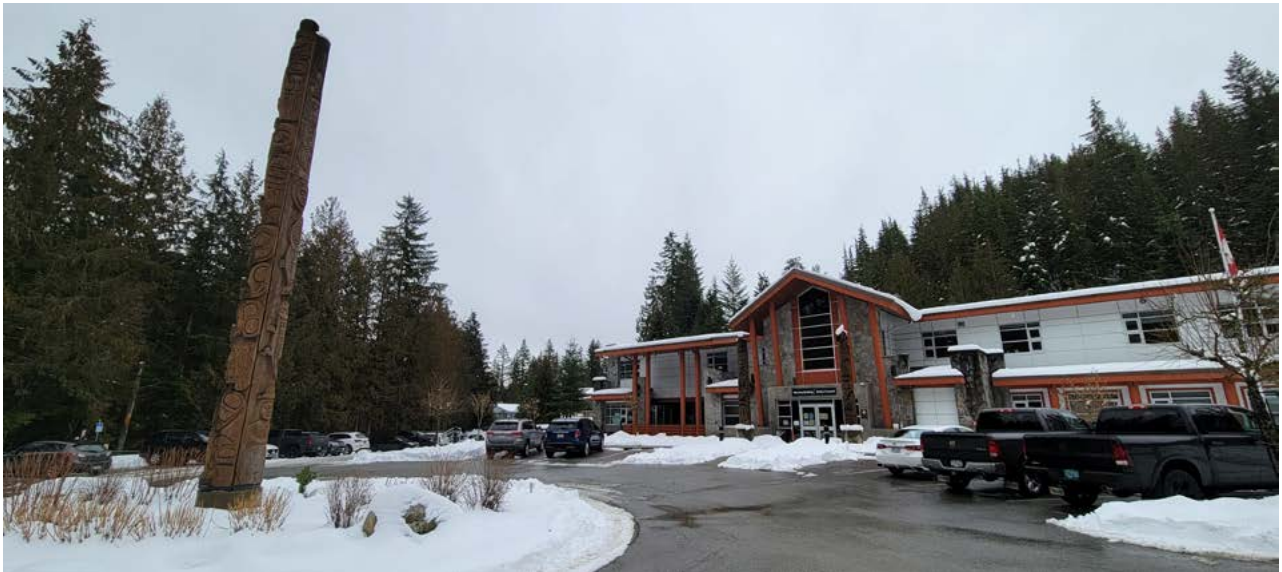
The Kwikw̓exwelhp Healing Village building (a CSC operated Healing Lodge).
